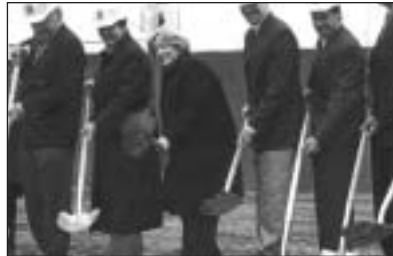
Breaking-ground for the new 221-unit, 17-story building going up at 415-21 W. Howard are Evanston officials with building developers and contractors of the highrise. At left is Bill Walsh, president of the developer, Bristol Chicago. To his right are Evanston Mayor Julia Walsh, and Ann Rainey, Alderman of the 8th Ward.
